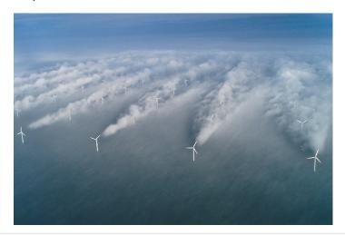
The photograph of off-shore turbines is the best photo I've seen that shows the airflow changes caused by turbines. In this case, note the downstream turbines, they're generating significantly less electricity being in the slowed wind.
