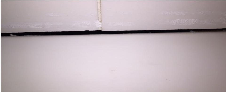
The contract reads: “NHCRS SERVICES, LLC WILL PERFORM THE FOLLOWING SERVICES IN THE TUBS/SHOWERS OF TWO BATHROOMS. REMOVE STICK ON CAULK APPLIED BY CLIENT. NHCRS SERVICES, LLC WILL FILL CAVITY BETWEEN BASE/TUB AND TILE/SURROUND WITH MORTAR MIXTURE SUFFICIENT TO BACK NEW CAULK APPLICATION. NHCRS SERVICES, LLC WILL APPLY NEW CAULK BEAD. NHCRS SERVICES, LLC WILL SUPPLY ALL MATERIALS AND DISPOSE OF DEBRIS.”
